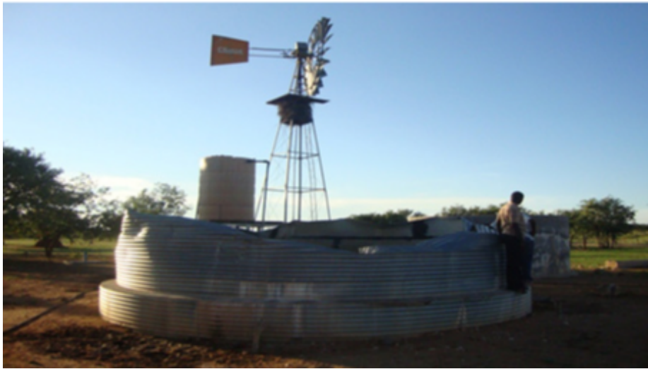
Image 15. Water tank destroyed by elephants. Photo: © John Mfune, March 2010, Mfune et al. 2013, p. 19.
